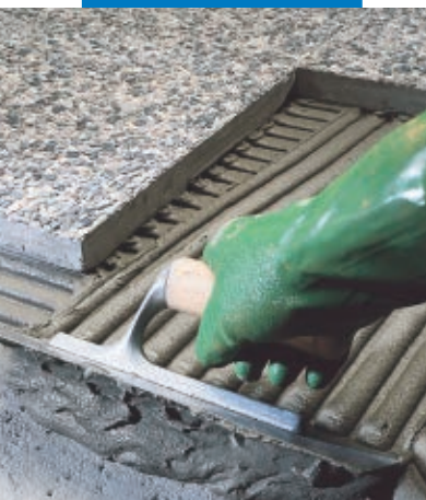
External installation of relief terrazzo "graniglie" tiles
