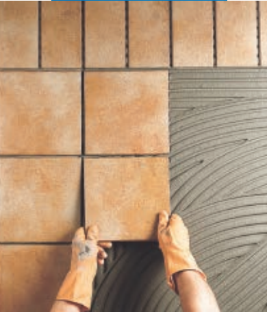
External installation of klinker tiles
